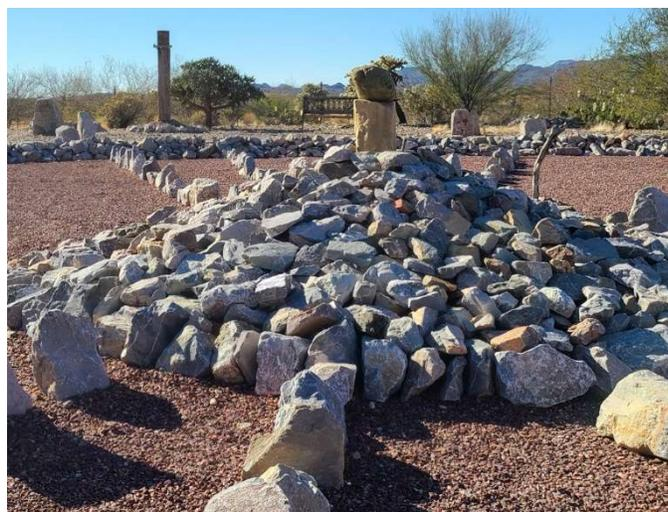
Next came the Sun Wheel's floor, "This step called for 28 ton of crushed decomposed granite <math><1/2</math> inch (1.25 cm) with fines (dust and dirt). Standard landscape material for southern Arizona. This was delivered and dumped inside the ring in 2 piles. The skid steer operator, in less than an hour had the granite looking like burgundy pile carpet, beautifully level and consistent."
