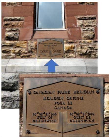
Fig. 10. Dominion Transit Circle Window and Prime Meridian
