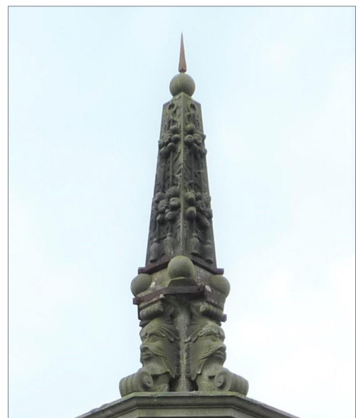
Fig. 12. The finial complete with ball and needle of the Newbattle right-hand sundial.
