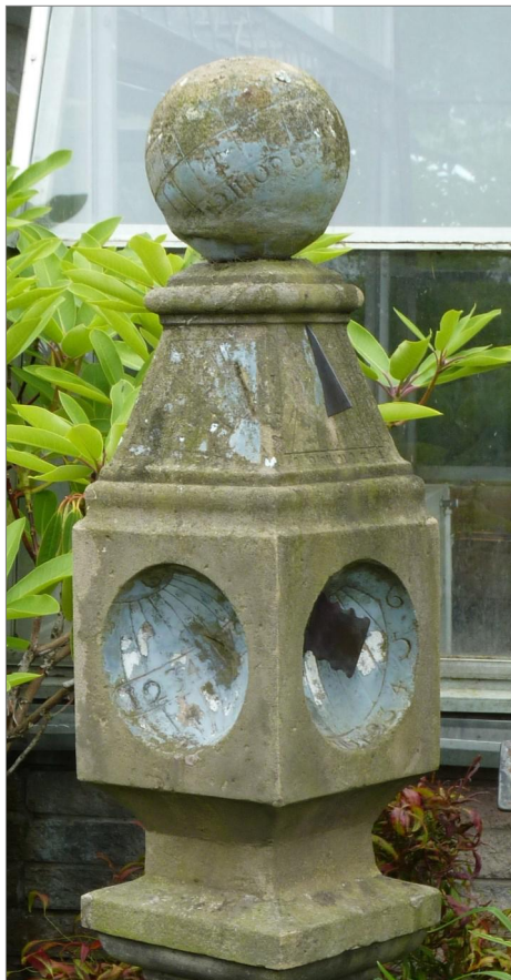
Fig. 18. The south face of the Duthie Park dial with the incorrect gnomon on the sunken dial face.
