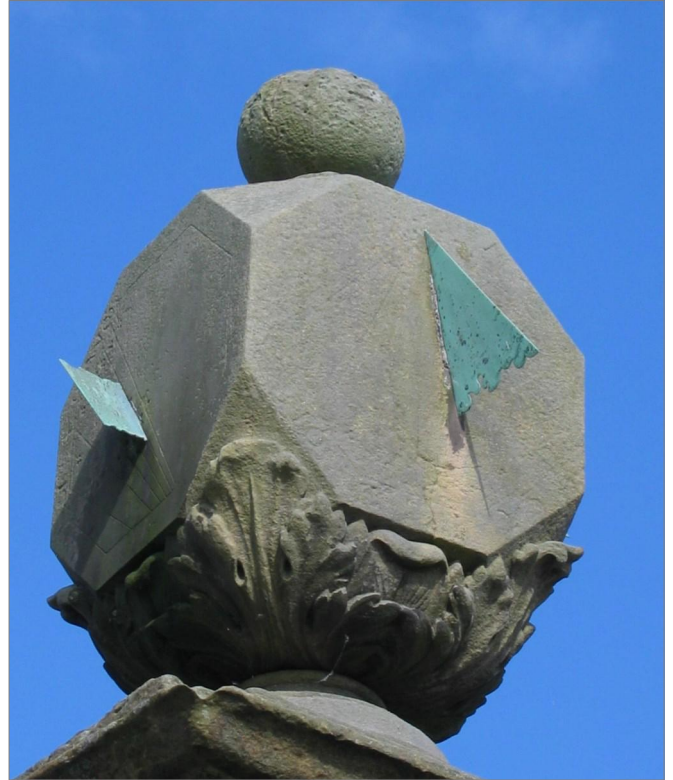
Fig. 10. Kinross House's right-hand sundial (viewed from outside the walls) showing the declining south and west faces.
