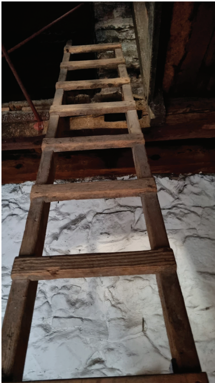
Fig. 5. The old wooden ladder giving access to the tower.
