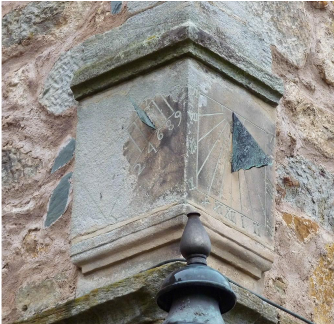
Fig. 8. Detail of the south and west vertical dials.
