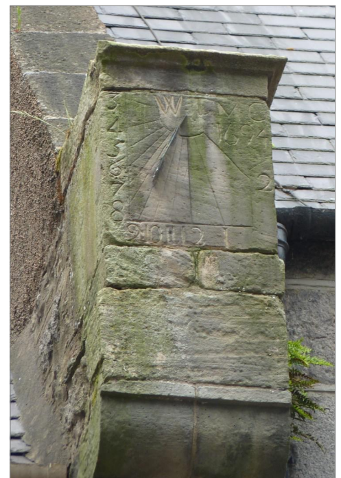
Fig. 8. The south-east face of the right-hand sundial at Upper Kirkgate.
