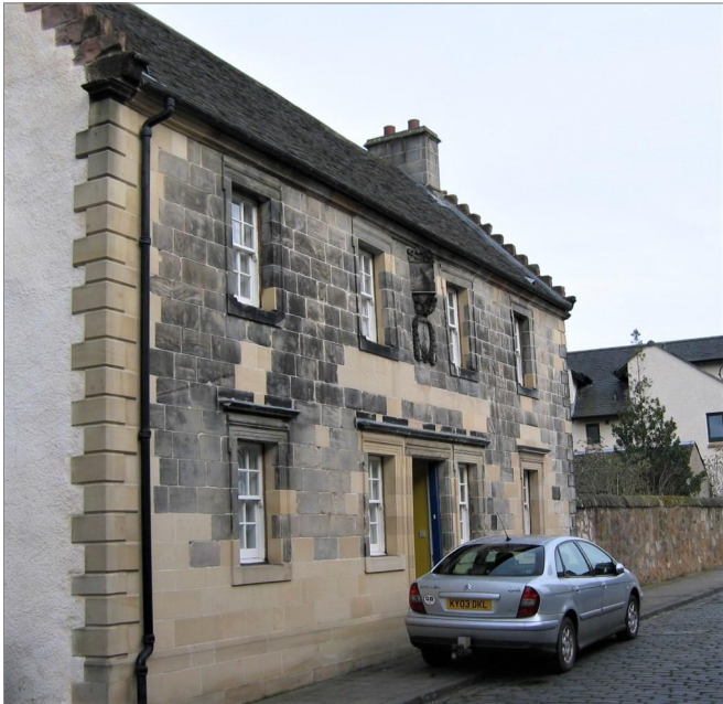
Fig. 12. The house in the Kirkgate, Alloa with the sundial in the centre of the upper storey.
