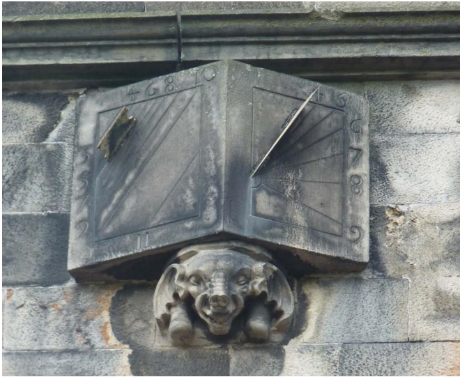
Fig. 14. Heriot's east-facing outside wall dial with elephant's head support.
