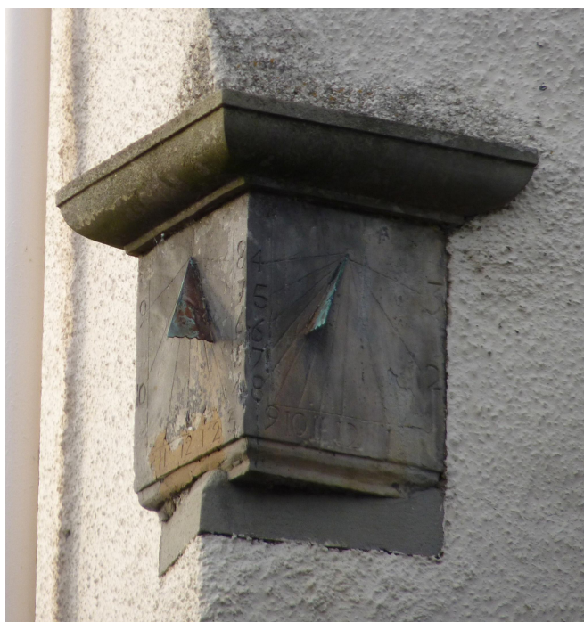
Fig. 3. Detail of the Dunnikier House / Path House dial.
