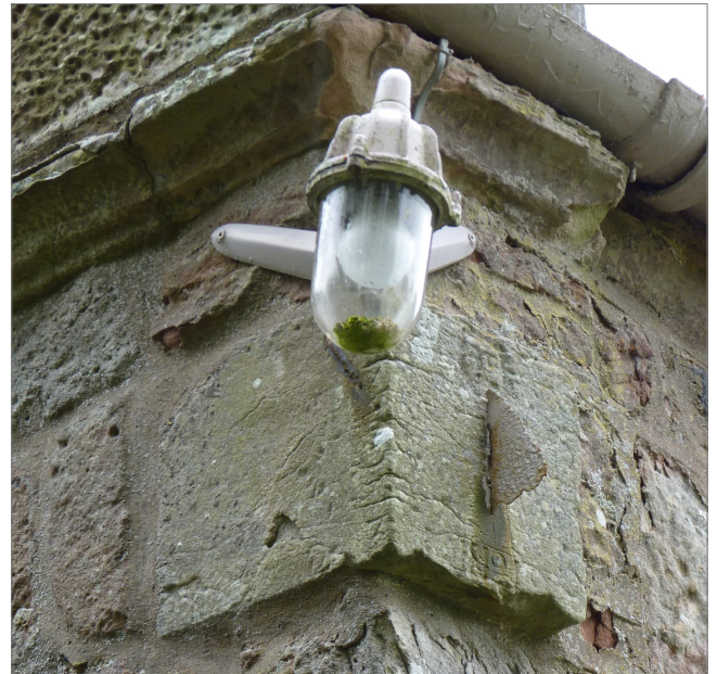
Fig. 6. The poorly positioned lamp above the Smailholm sundial. Both faces are in very poor condition.
