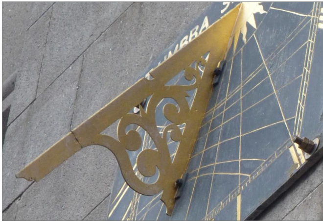
Fig. 4. Close-up of the Town House gnomon showing the nodus and the repair.
