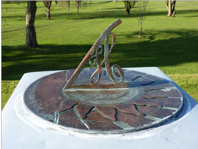
Fig. 14. The rather fine “H” for Halkett supporting the gnomon.
