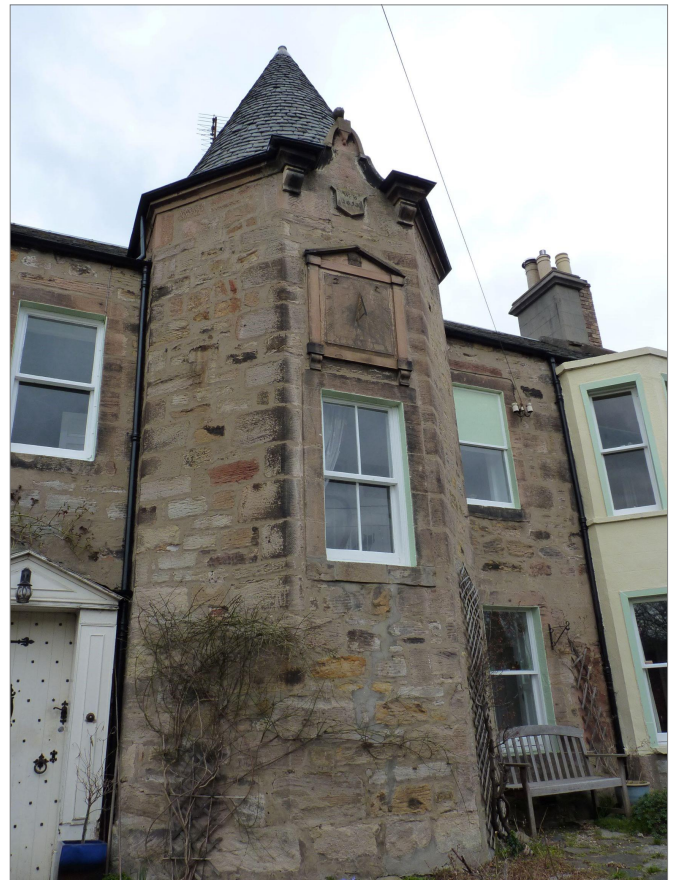
Fig. 10. The Dalkeith sundial showing its position above the first floor window of the tower.
