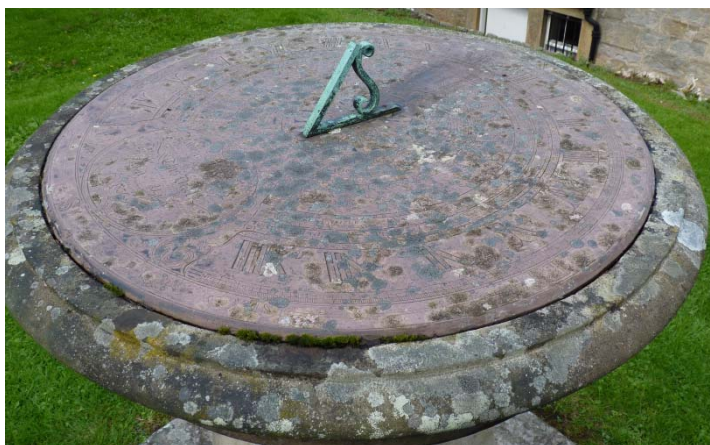
Fig. 4. Detail of the Currie dial plate, with missing gnomon tail.
