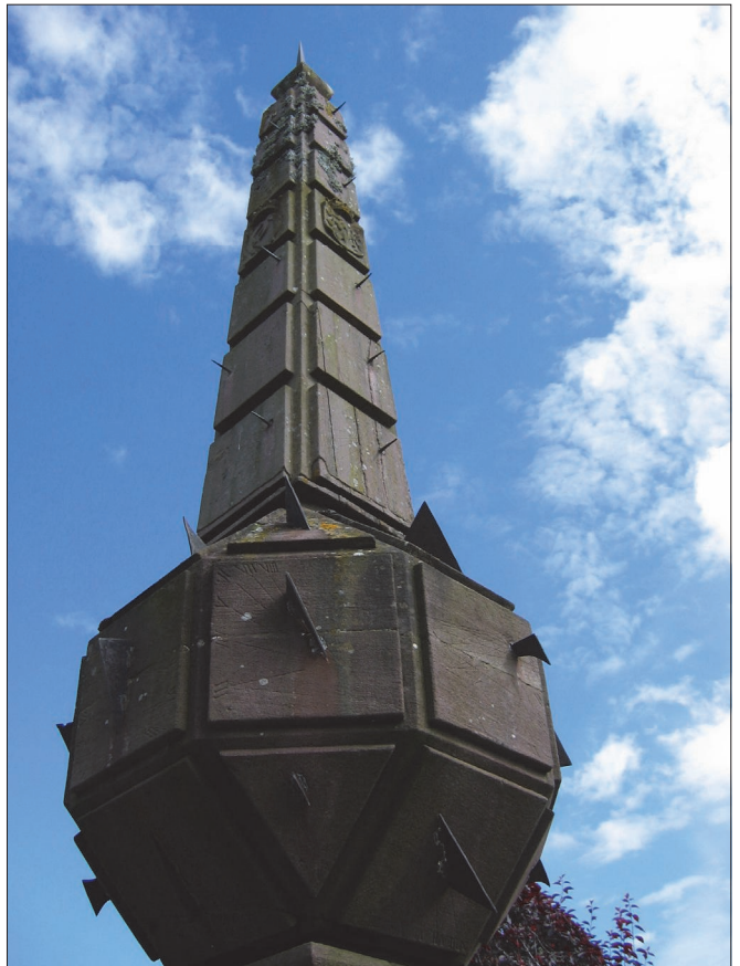
Fig. 6. The boss and finial of the Drummond Castle dial. Most of the individual dials still have their gnomons in place.
