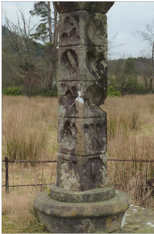
Fig. 14. The damage on the middle section of the shaft of the Asknish obelisk.
