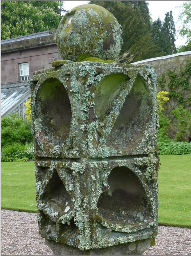
Fig. 12. The step on top of the Brechin shaft which would not be present on an obelisk sundial.
