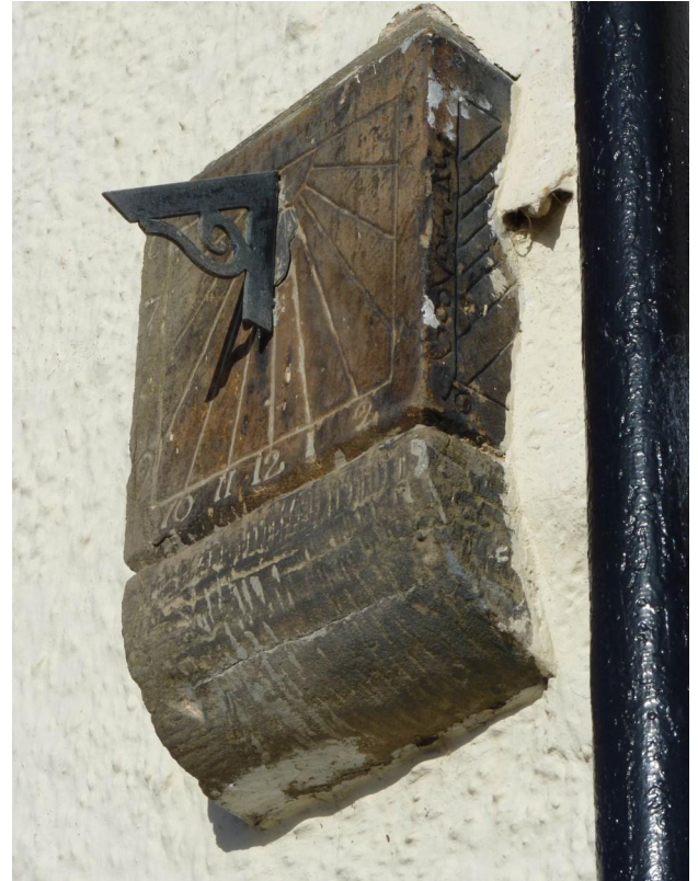
Fig. 6. The east face of the second Limekilns sundial significantly covered by the addition of the harling.
