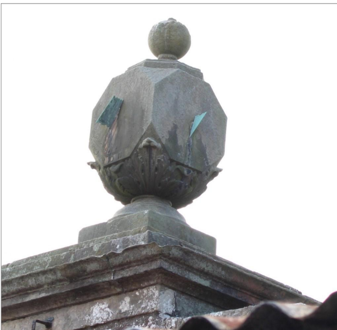
Fig. 9. Kinross House's right-hand sundial (viewed from outside the walls) showing the declining north and east faces.
