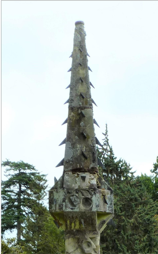
Fig. 17. The finial's north face of the Mount Stuart obelisk on the left side with the incorrect gnomons.
