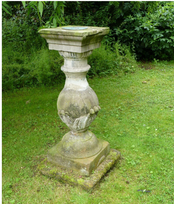
baluster support with boldly cut egg and dart enrichment supporting a square abacus, on which is placed the bronze dial-plate."
