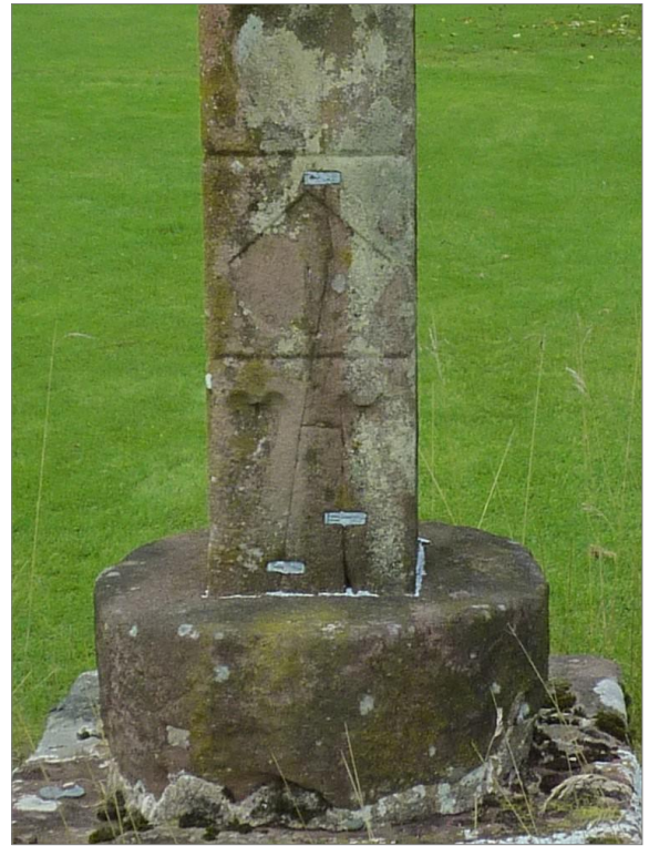
Fig. 4. The cracks in the Ballindalloch shaft held together with metal ties.
