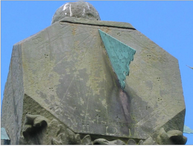
Fig. 8. Detail of Kinross House's left-hand sundial (viewed from outside the walls) showing the declining south face.
