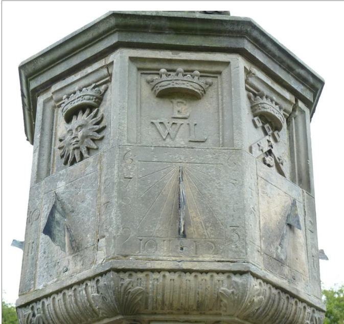
Fig. 9. The south face of the Newbattle right-hand sundial and the adjacent south-east and south-west faces, with the dials and decorated spaces above them. Note the huge crack near the top of the south-east face.
