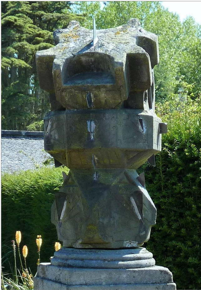
Fig. 15. View showing the north faces and the star on top of the Culzean Castle sundial.
