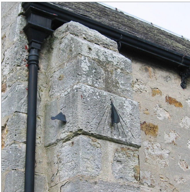
Fig. 4. The south and west faces of the dial on the south-west buttress of Pencaitland church.
