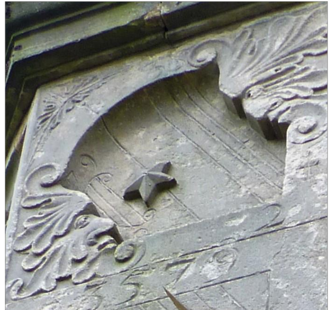
Fig. 6b. Close-up of the sunken west-facing dial-pair with its two gnomons and two sets of hour lines.
