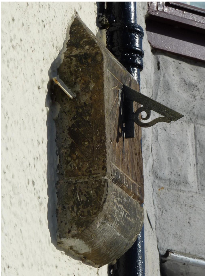
Fig. 5. The west face of the second Limekilns sundial partly covered by the addition of the harling.
