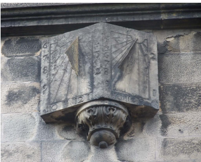
Fig. 16. Heriot's south-facing outside wall dial.
