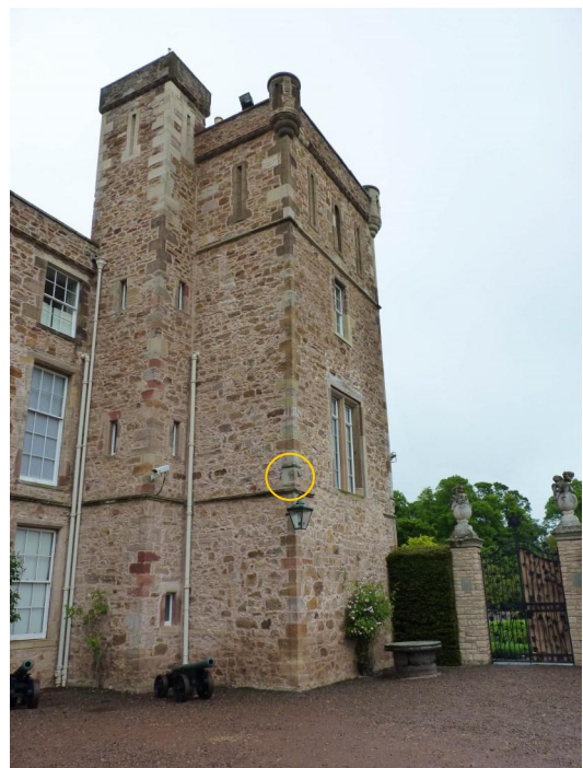
Fig. 7. The south and west vertical dials (circled) above the lamp on the corner of the house.
