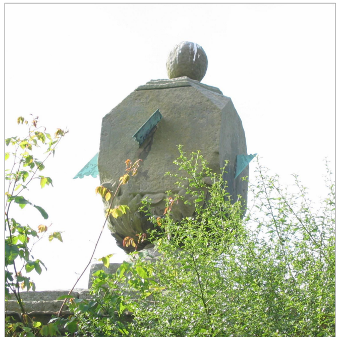
Fig. 7. Kinross House's left-hand sundial (viewed from outside the walls) showing the declining east face.
