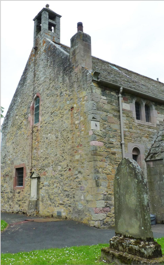
Fig. 13. The dial at the south-west corner of Bowden Kirk with the skew-stone above. The external bell rope, a common feature of many 17th-century Scottish churches, can also be seen.
