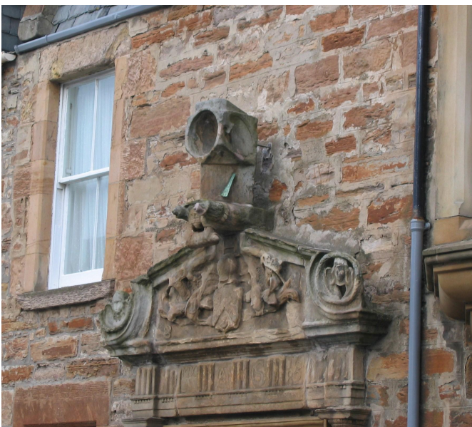
Fig. 9. The top of the Muckle Yett doorway today.
