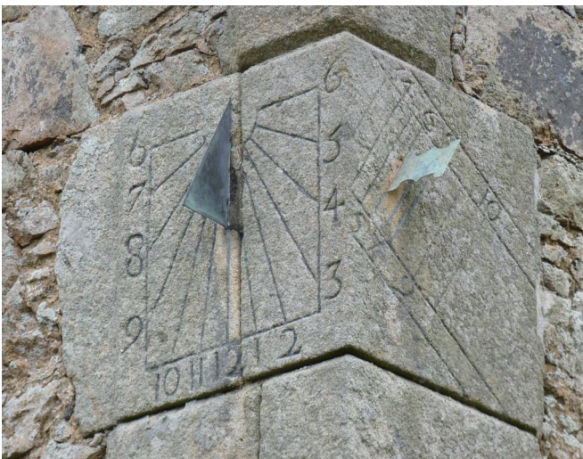
Fig. 15. The south- and east-facing dials with the wrongly positioned gnomon on the south face.
