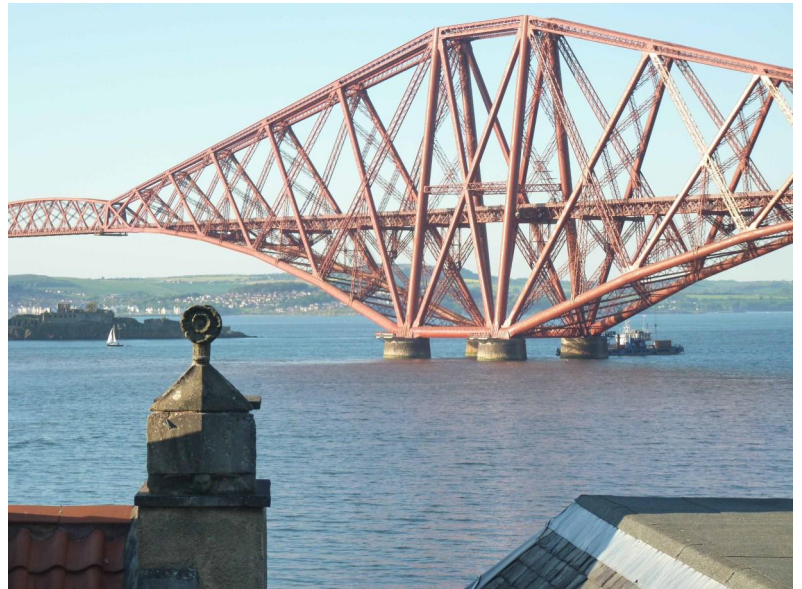
Fig. 30. South Queensferry dial showing altered roofline.
