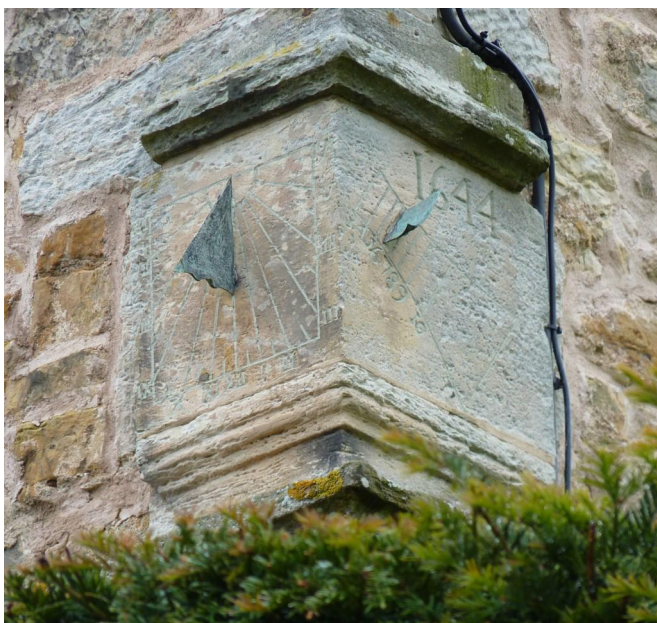
Fig. 5. The south and east vertical dials today with the probably re-engraved date.
