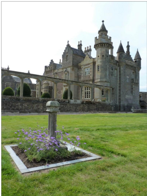
Fig. 16. The pedestal of Sir Walter Scott's sundial. The horizontal sundial has been missing for many years.
