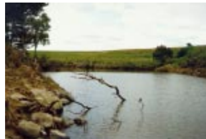
A scour hole containing a salt pool on the Barwon river in Victoria, Australia.
