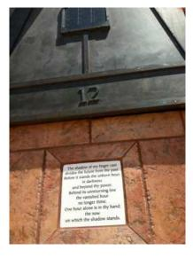
The gnomon (the 'g' is silent) must point toward true north in order for the sundial to work. Other calculations must be made to determine the angle that the sundial must face for its specific latitude and longitude.
