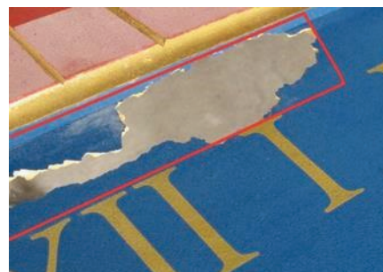
Fig. 2. The dial in 2014. Left: Squirrel entering nest via hole in face of dial. Right: Detail of the damage.
