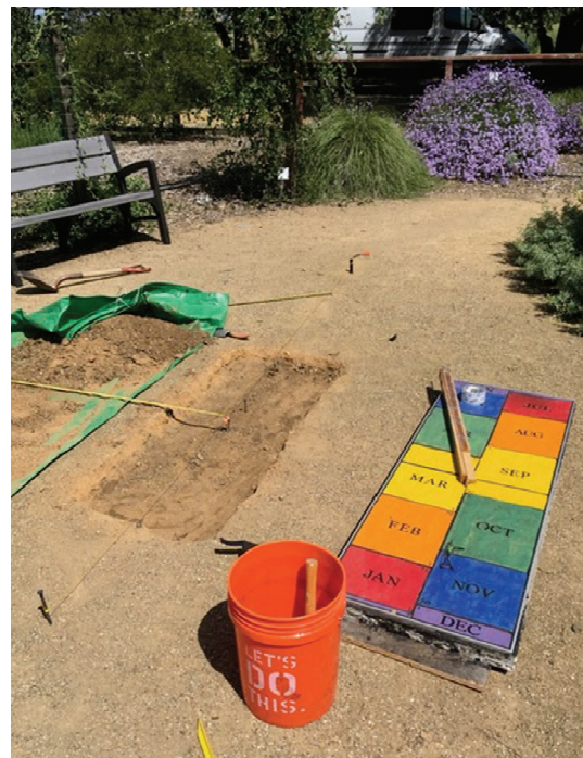
Fig. 5. Hole dug for declination scale with N-S and E-W lines marked.
