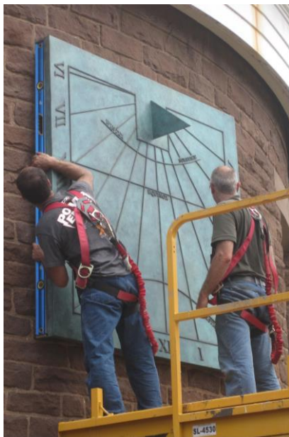
Fig. 10. Plumbing and leveling the dial.
