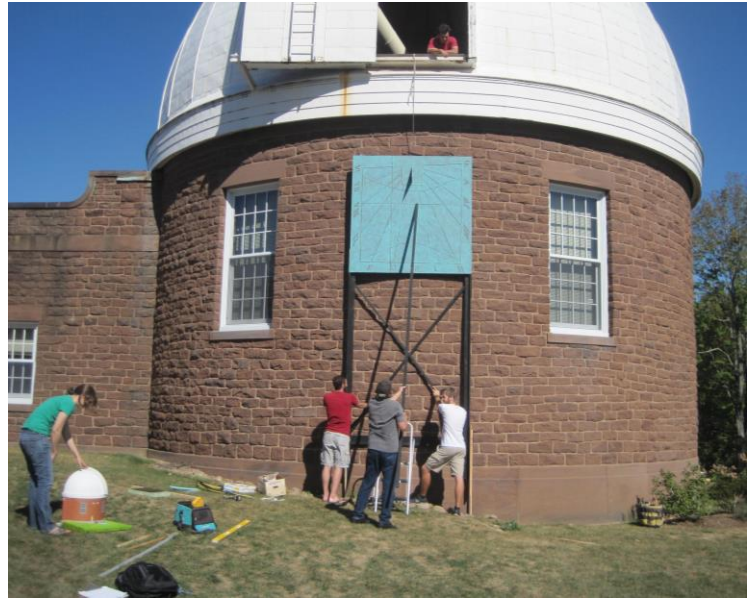
Fig. 4. Field testing the mockup on the building.
