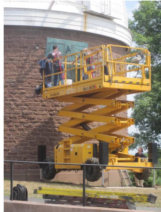
Fig. 9. Positioning the dial on the curved wall.
